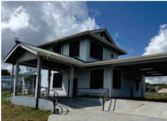
GLSC Port Kaituma Sub-Regional Office, Administrative Region 1, Barimi-Waini
